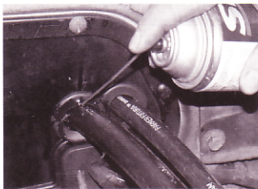
11. Benny decided to run the A/C hoses to the cooling unit from the driver's side so two holes were drilled in the firewall, grommets were fitted and the hoses slipped into the cabin. (Note-A spray lubricant makes it easier to push the hoses through.)
